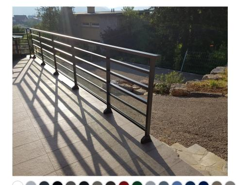
The Ted guardrail features sleek, modern lines that ensure safety and solidity. Its 44.2 laminated glass ensures maximum strength thanks to the different layers held together by a PVB filter, which keeps the pieces of glass together in the event of glass breakage. A safe choice that suits all tastes and styles.
